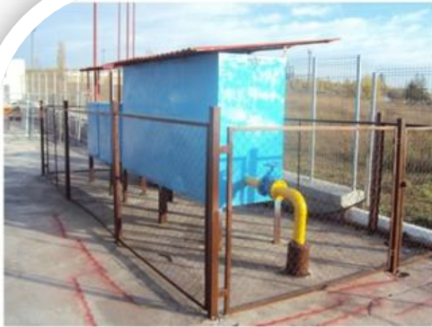
Gas distribution point
