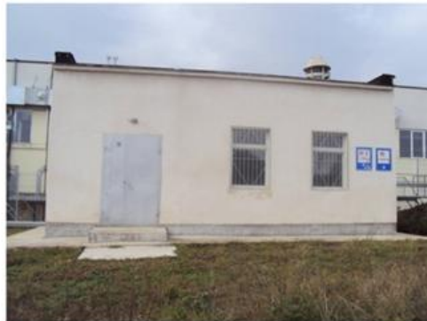
Pumping stations with anti-incendiary reservoirs for the whole complex
