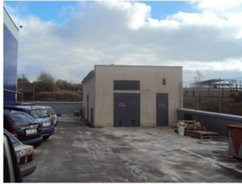
Power distribution station
