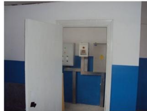
Pumping station control point
